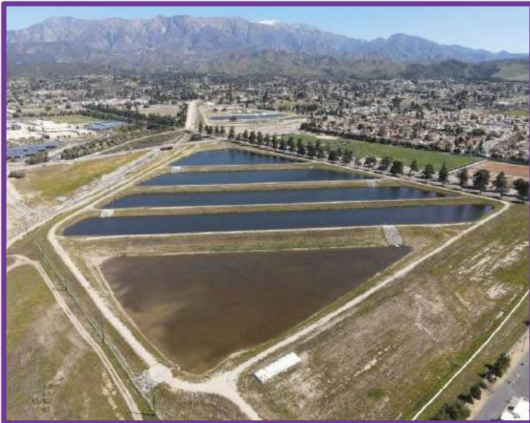
Brookside East Recharge Facility
