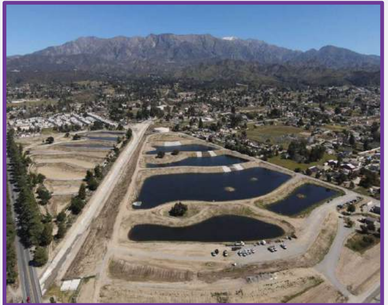
BCVWD Recharge Facilities
