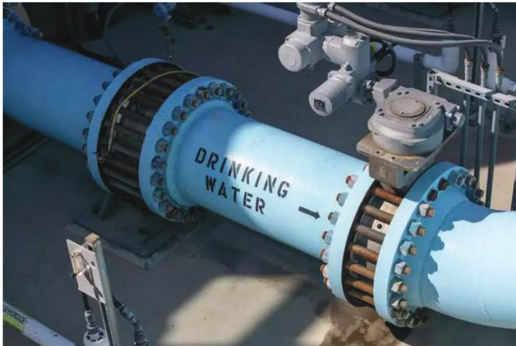
A view of a water pipe in the post-treatment section, which includes adding minerals and disinfecting with chlorine, at the Claude “Bud” Lewis Carlsbad Desalination Plant, on March 30, 2022, in Carlsbad, Calif.
