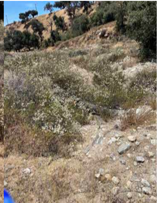
Pipeline to be Abandoned - SW View
