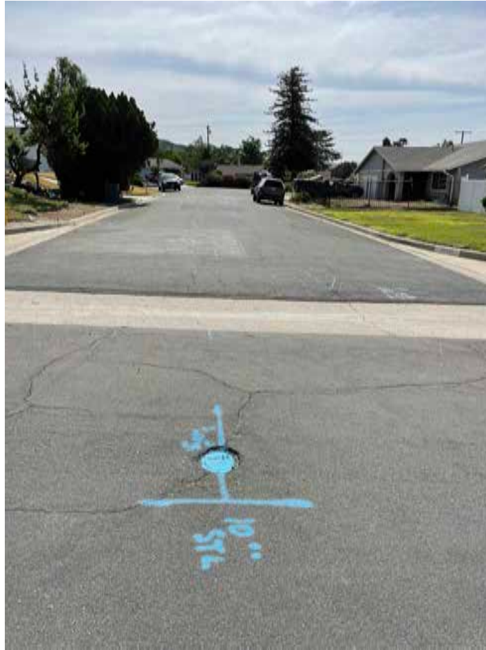
East View of Bing Place
