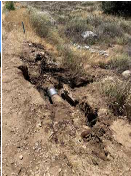
Pipeline to be Abandoned - SW View
