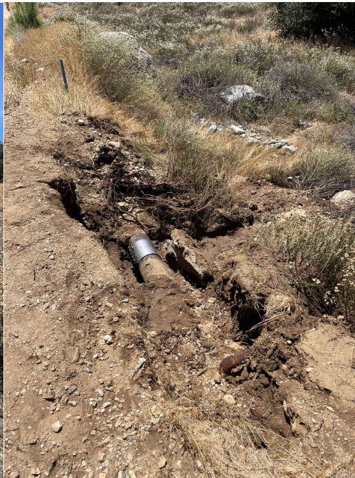
Pipeline to be Abandoned - SW View
