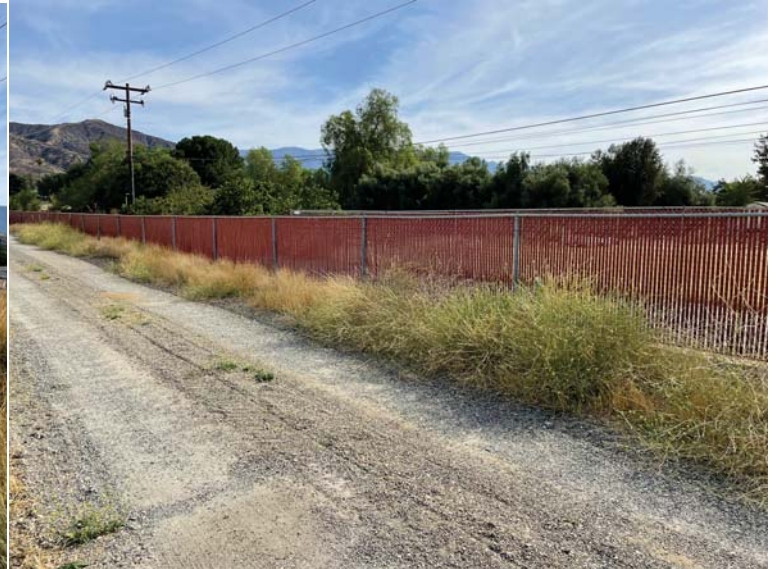
Northeast View of Pipeline Alignment
