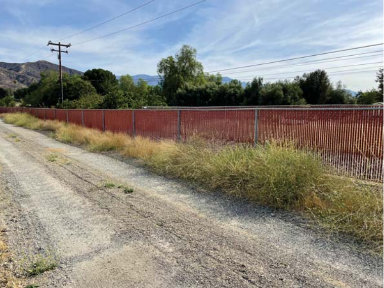
Northeast View of Pipeline Alignment
