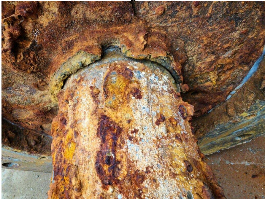
Photo 2 Highland Springs Booster Pumping Unit Column to Discharge Head Connection
