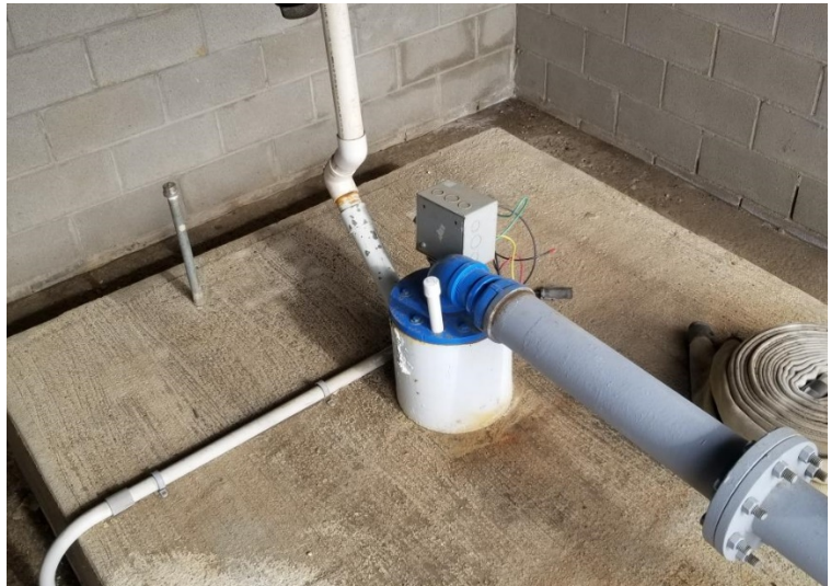
Well 10 Discharge Piping
