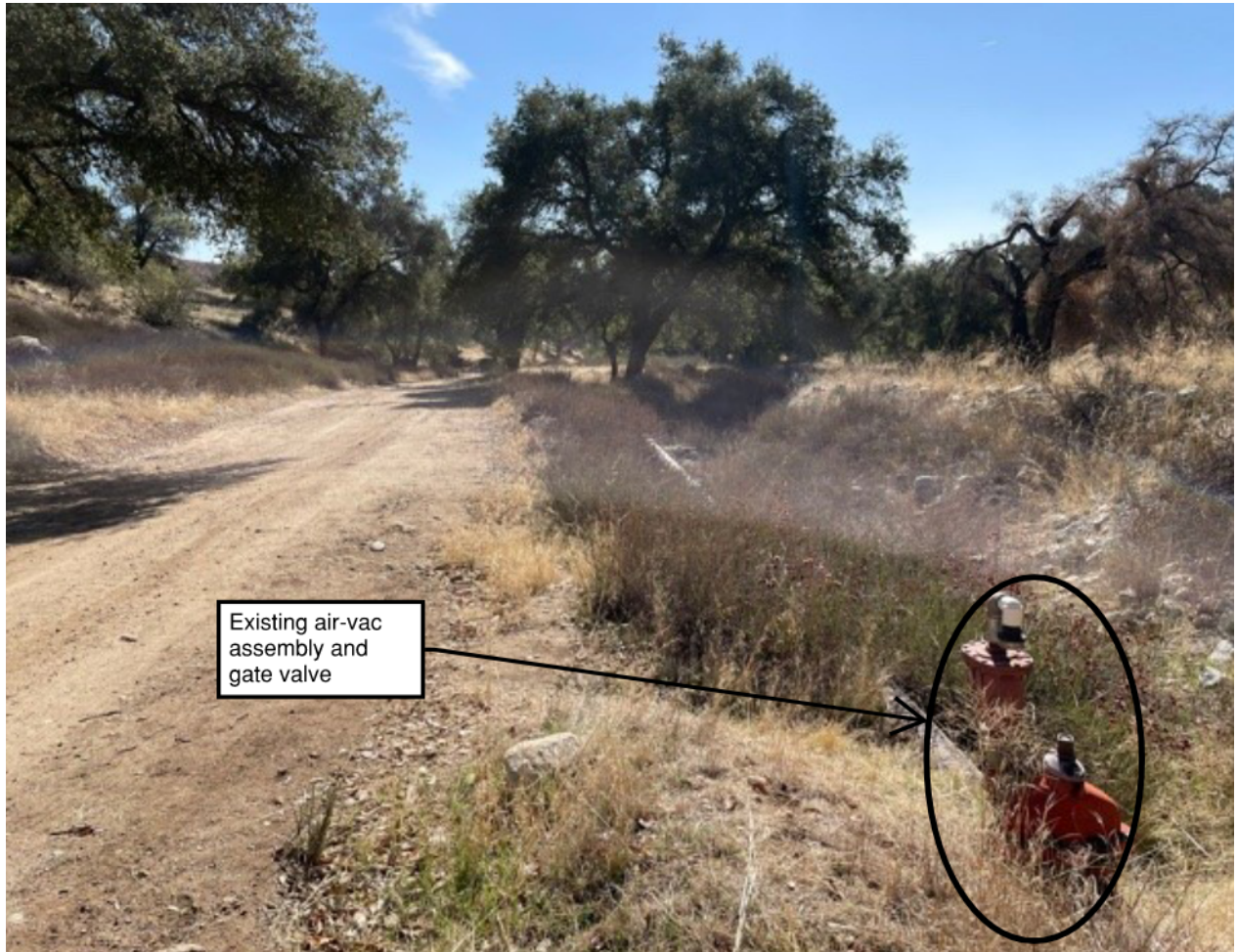
Figure 5 – Existing Waterline Appurtenances
