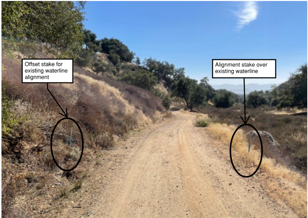
Figure 4 – Typical Existing Waterline Location Staking
