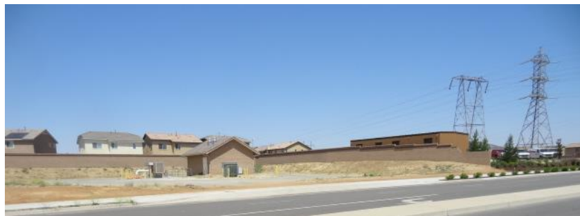
Well 25 Facilities from Starlight Ave Looking West
