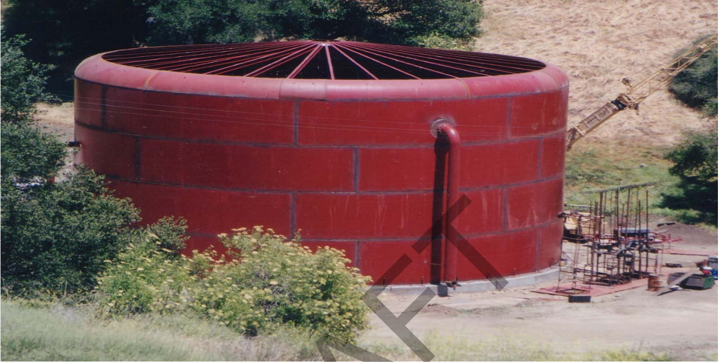
The Upper Edgar Reservoir, seen here under construction, was built in 2000.
