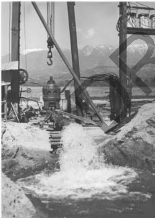
Well 1 is seen here being flushed for the first time in 1935. Well 1 is located at the intersection of 12 th and Palm but predates the surrounding structures
