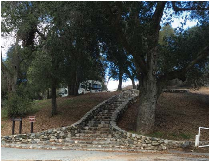
Cobble stairs in good condition, but sediment/erosion issues on the road below.
