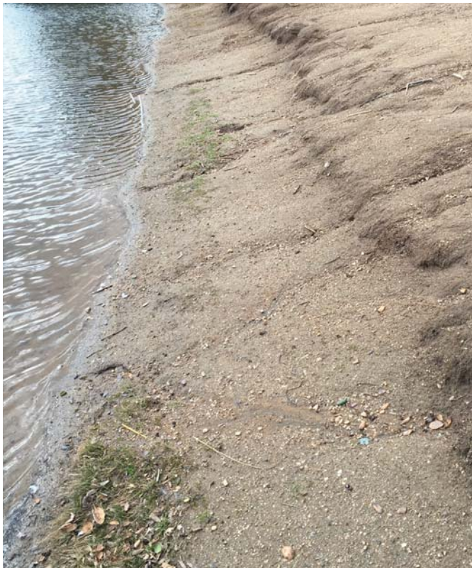
Erosion into the pond.
