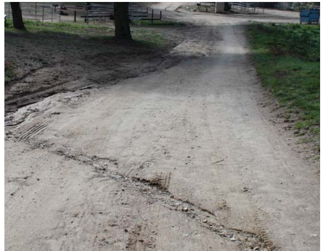
Erosion/drainage issues along the dirt roads.
