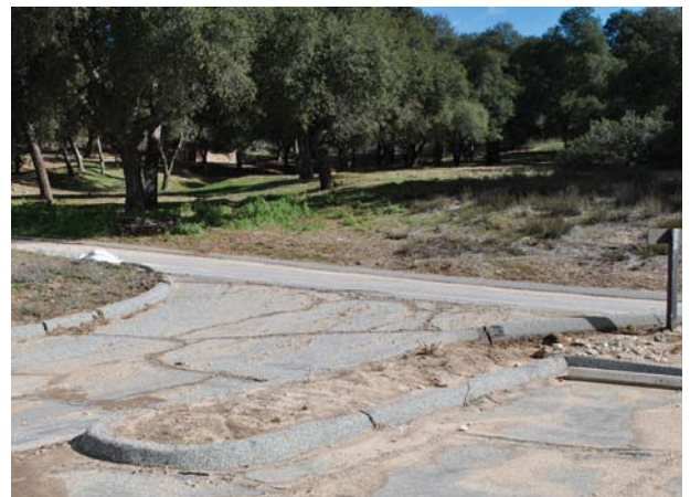
Example of the pavement and curb with erosion control repairs that are required.
