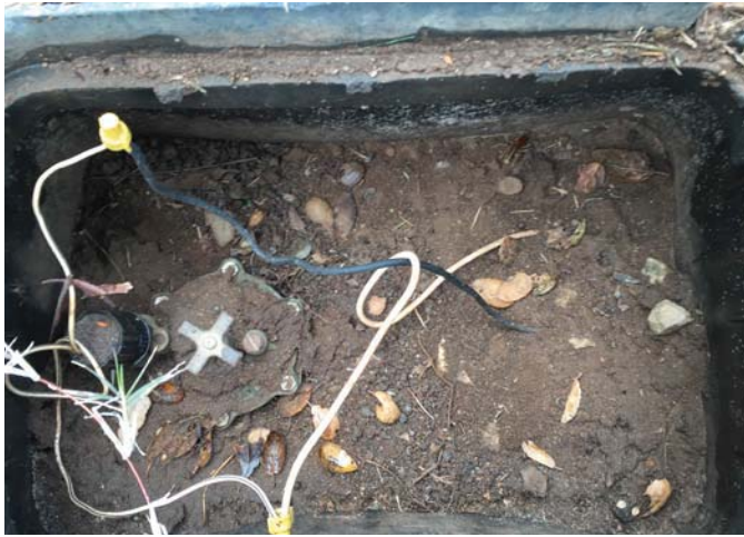
Sediment filled irrigation control box.
