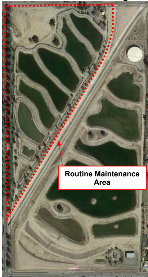
Figure 2 Site 2 – Noble Creek Recharge Facility Phase I
