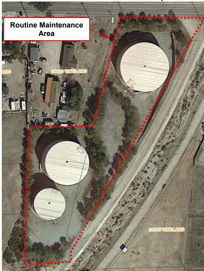
Figure 16 Site 16 – 2850 Pressure Zone Reservoir (Vineland Tanks)
